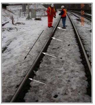
**Photo 1b.** Mile 0.06 of the Dundas Subdivision. The black arrow shows the direction of train movement. White arrows point to impact marks on the gauge side of the south rail, south track.
