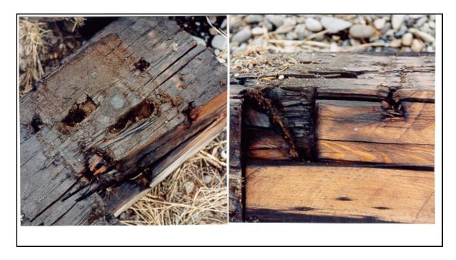
the rails. Figure 4 shows the lateral movement at the spike hole.
