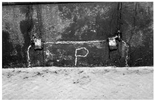
The effective height of the port and starboard side bulwarks within the superstructure was 0.91 m, while that in way of the chain rails at the open after end of the main deck was 660 mm.
