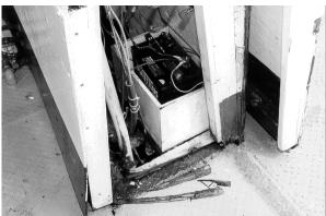
The deteriorated condition of the inboard edge of the wooden frame in way of two of the three hinges of the bridge front door was such that the holding power of the 25 mm long screw fastenings was markedly reduced. The timber and wood packing in way of the hinge screw holes was decayed such that the screws were pulled clear with the door. The third and lowest door hinge remained attached to the door frame, and its screw fastenings were pulled clear from the door itself.
