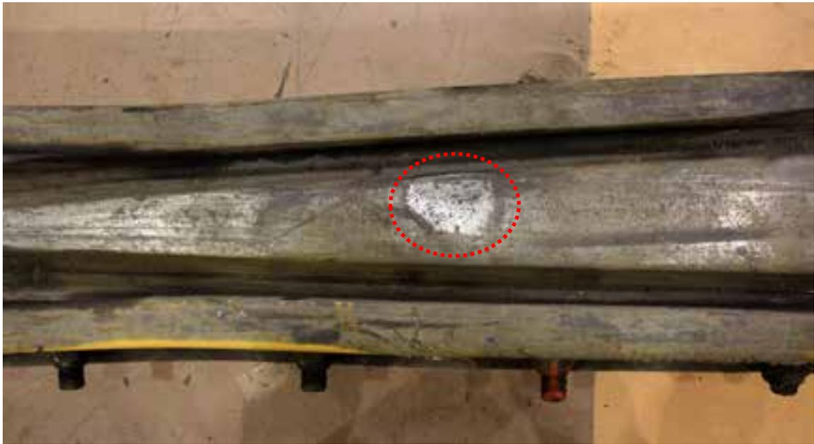
Figure 7: Weld repair on the frog about 3.5 feet from the point tip
